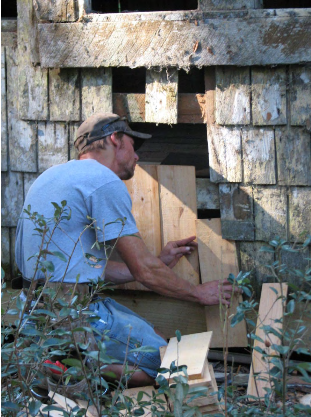
(2011_02_22, IMG 4856) Care was taken at every step of the process by Jeff and each of his crew. This is evident while viewing Shane Campbell carefully weaving in a replacement shingle among the original siding.
