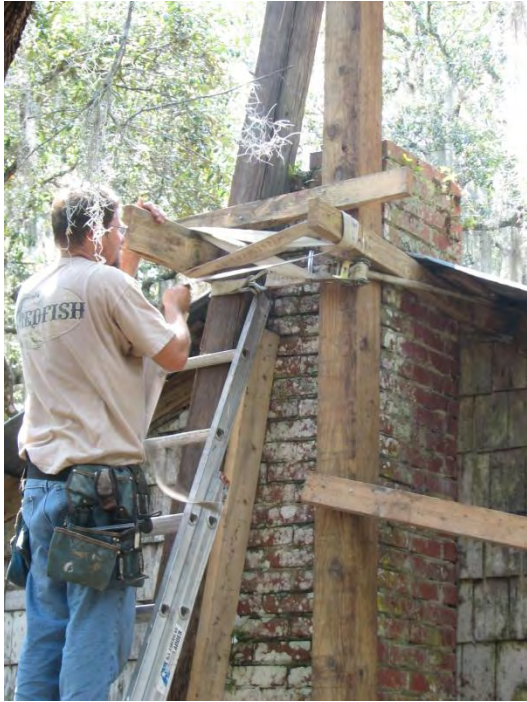
Jeff Penuel secures timber “strong-backs” to chimney prior to “righting”. (2009-06-09, IMG 3558)
