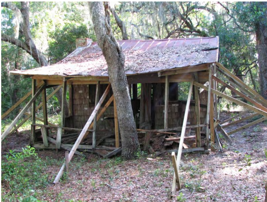
Initial bracing of cabin in 2007. (2007-07-11, IMG 1215)
