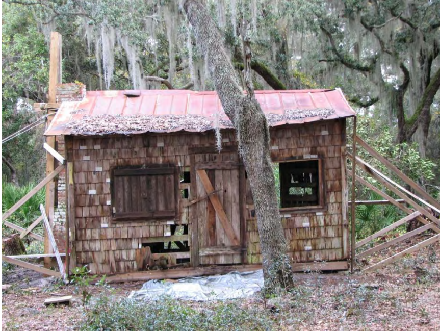
Cabin with straightened chimney. Note top right corner having moved ca. 8-10" from the released bracing to achieve level. Jeff intentionally incorporated the chimney wall in with his interior "strongbacks" for additional support, which allowed the structure to "right" itself, while still attached to the chimney. (2009-13-03, IMG4013)
