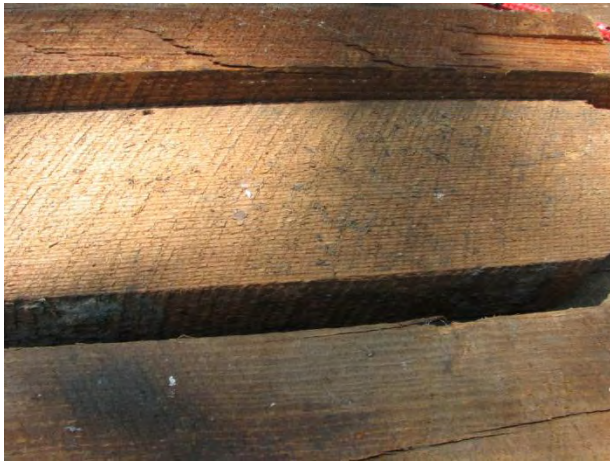
Close-up of lumber showing grain and old circular saw cuts-marks. (2010-07-09, IMG 4638)
