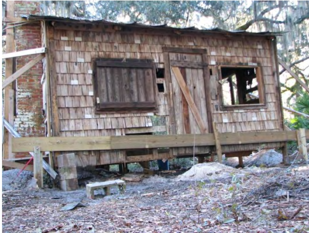
The “levitated” cabin, with foundation and subfloor removed! (2010-03-01, IMG 4252)
