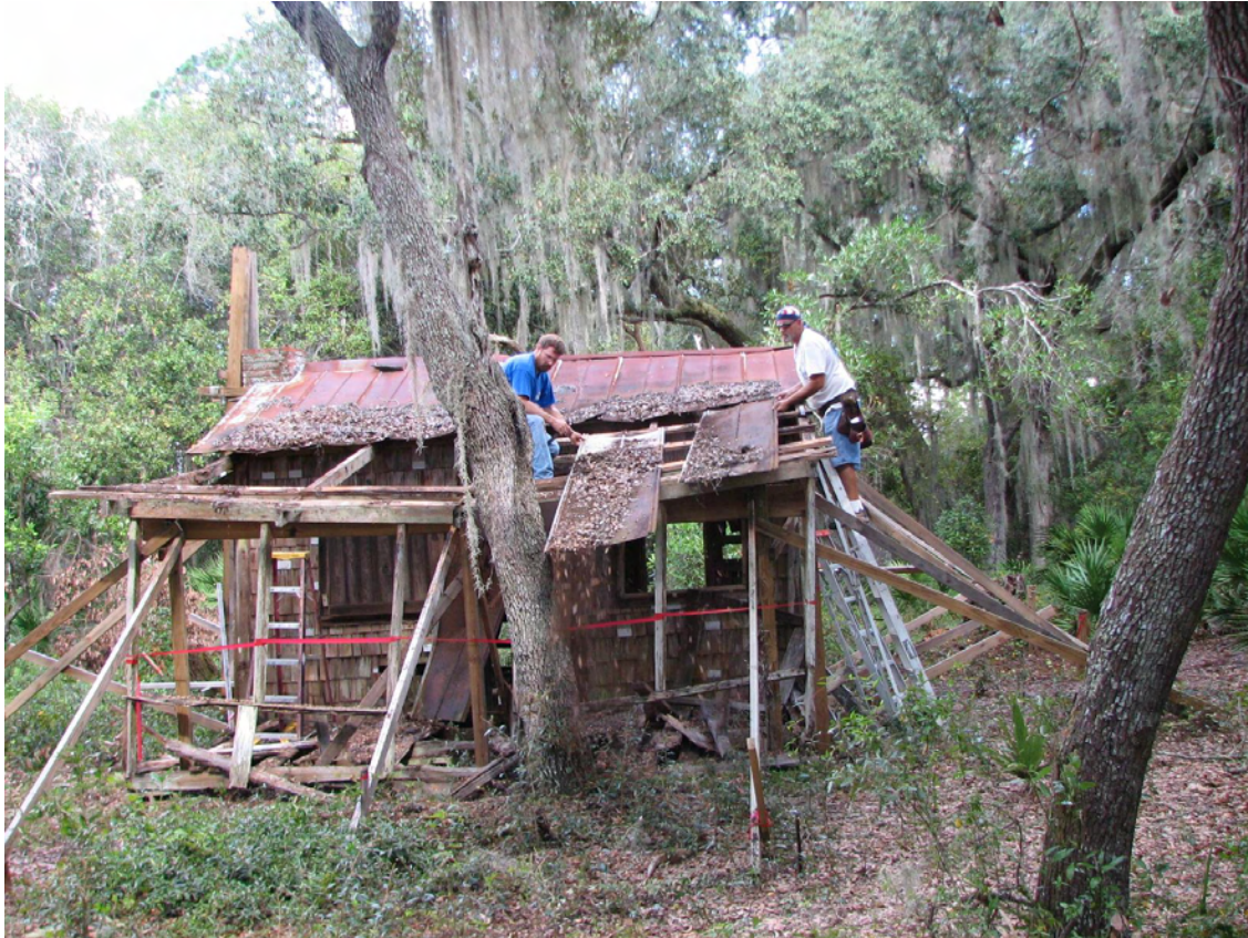
Careful dismantling of deteriorated portions of the cabin. (2009-10-29, IMG 3888)
