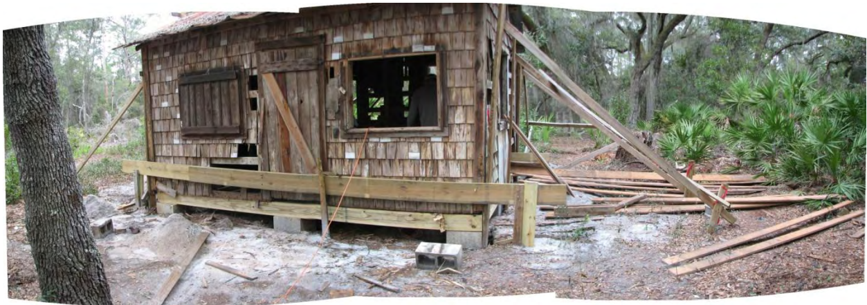
New foundation, sub-floor and original floor boards (on right) ready to re-install. (2010-03-17, IMG Carr Cabin Floor re-install)
