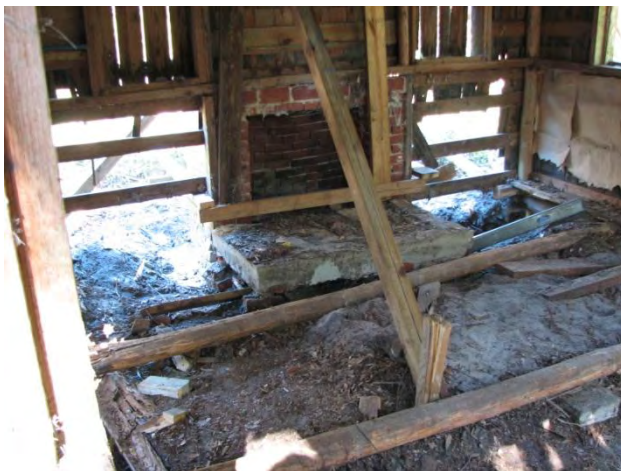
Hearth being leveled. (2010-01-19, IMG 4066)
