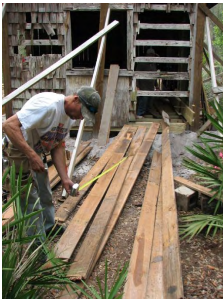
Inspecting and trimming rotten material from sound original floorboards. (2010-03-17, IMG 4396)
