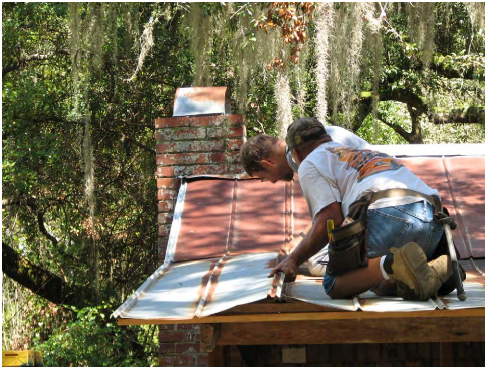
"Distressed" but sound tin fitted to porch roof. (2011-09-23, IMG 5463)
