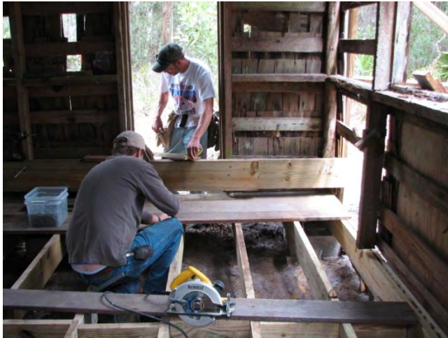
Re-installing “sound” original floorboards. (2010-03-17, IMG 4411)
