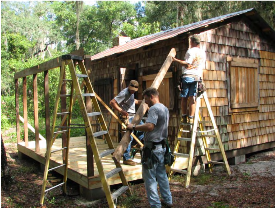
Porch framing going up utilizing the few surviving, sound timbers. (2011-09-23, IMG 5415)
