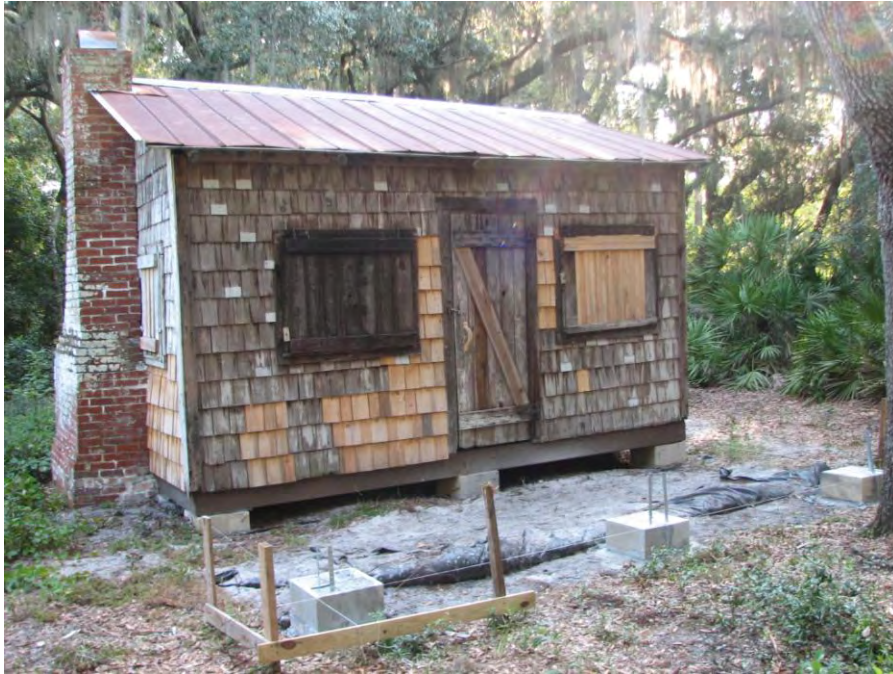
(2011_09_15), IMG5361) Concrete block porch piers laid and ready, 9-15-2011.
