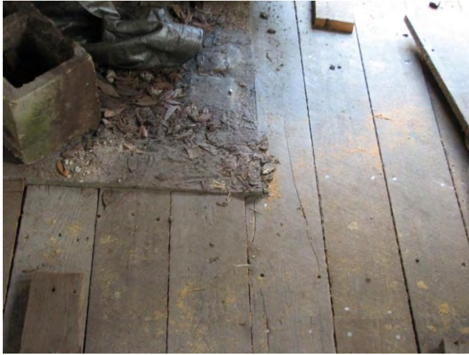
Re-installed, original floorboards, set to hearth elevation. (2010-03-18, IMG 4417)
