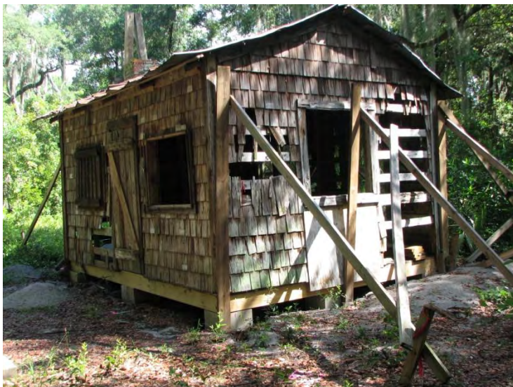
Cabin "de-levitated", with leveled chimney and restored floor set back down on a new and substantial subfloor and foundation...all to protocol. (2010-06-23, IMG 4597)
